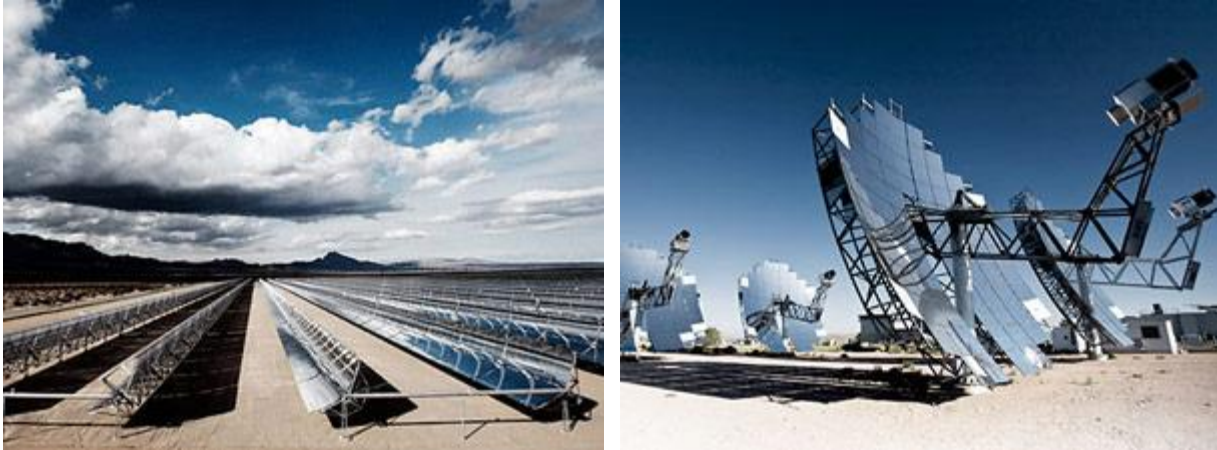
Figure 7 Parabolic trough and solar dish CSP (Hutchinson, 2008).
